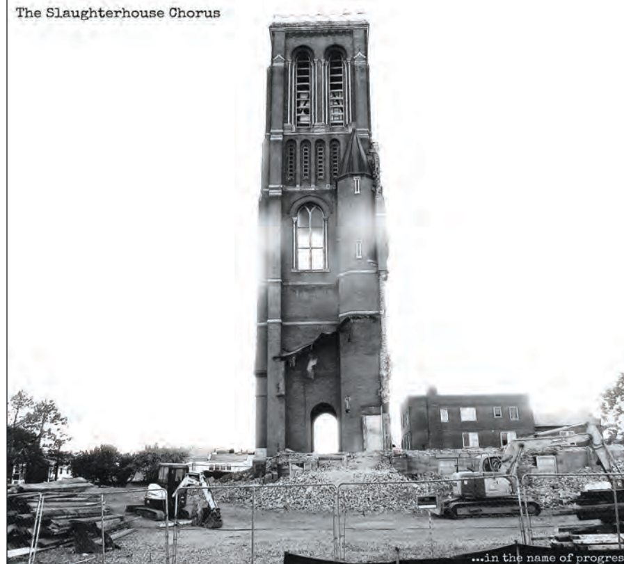
■ St. Patrick's Church in Watervliet during demolition
